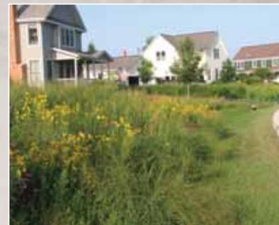
A bioswale along a residential street collects and filters stormwater runoff without curb and gutters.
