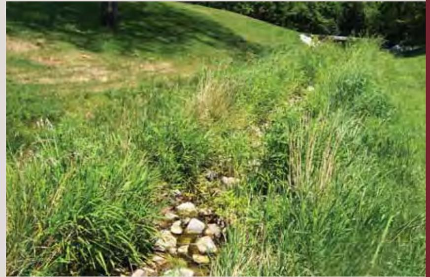
*A bioswale can effectively capture and direct rainwater runoff to specific locations while protecting your property. Simple design practices including grasses and sedges can be used, or more colorful flowering plants can also be established in the bioswale.*
