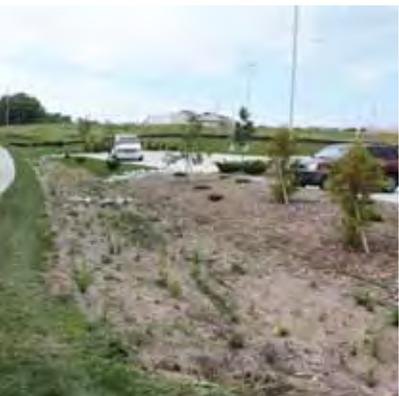
*This bioswale was recently planted along a park corridor and will direct water off of parking lots to a nearby storm drain while water is infiltrated into the soil as it moves along the swale.*
