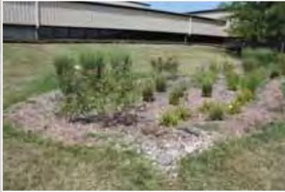
An example of reinforcement for the overflow of a school site rain garden. When the garden fills, it will overflow on the gravel rocks and not damage the remainder of the berm that holds the water in the garden.
