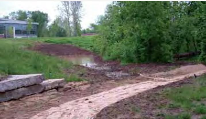
*The depth and construction of a bioswale often does not require substantial excavation or materials. Here a bioswale receives overflow from a new rain garden, and is protected by an erosion control mat until it is complete.*
