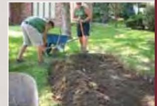
*Excavate and form the rain garden to the designed depth, and form berms on the downhill side (left).*
