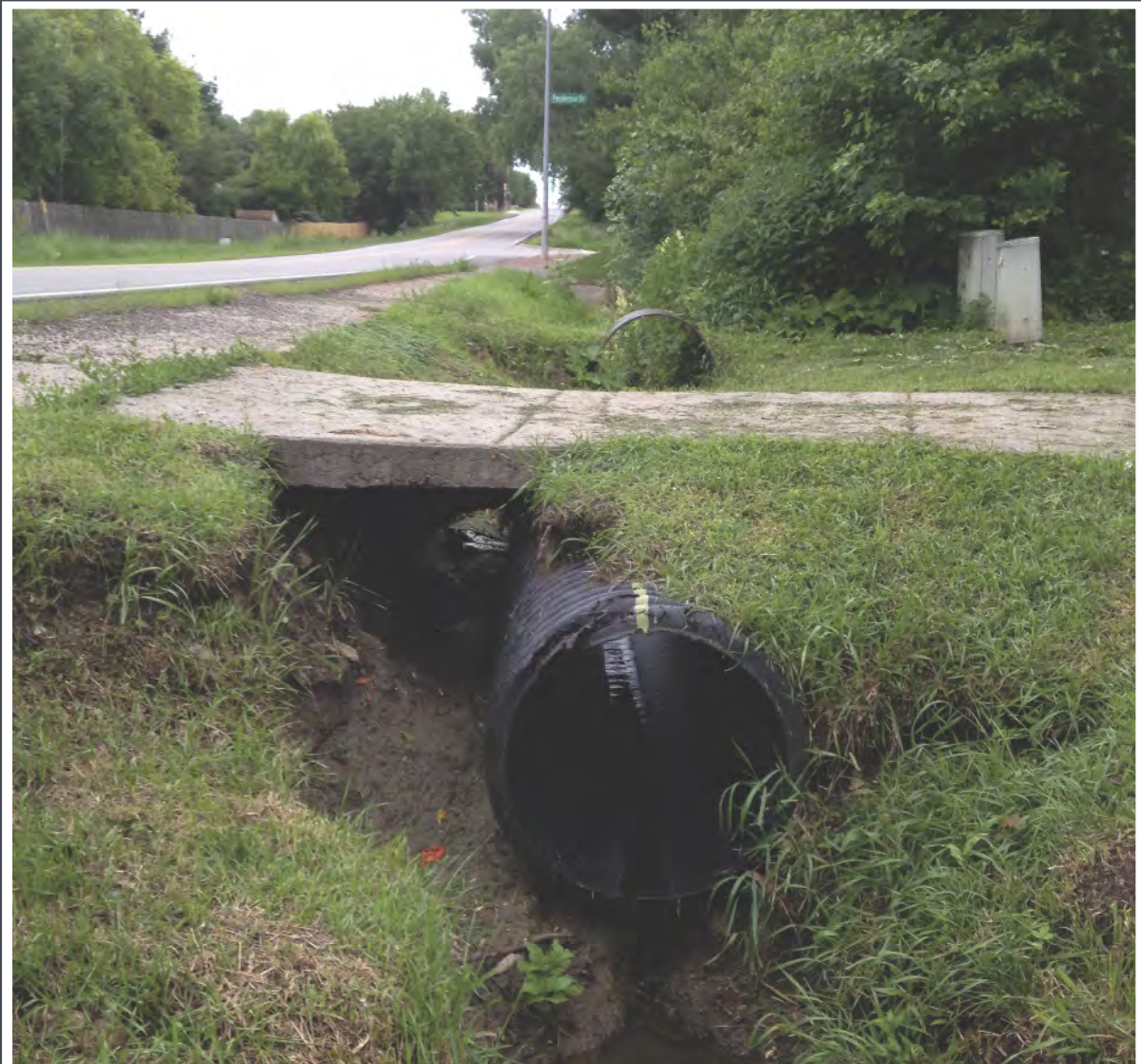
A roadside ditch unable to withstand the runoff being directed to it, creating multiple issues
