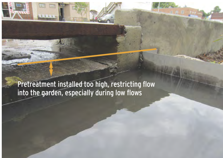
The 'curb-well' pre-treatment in this project was installed too high, creating backwater conditions that allow flows to bypass the garden, especially in low-flow events. The 'curb-well' should be installed with V-notch weirs or level with the pavement.
