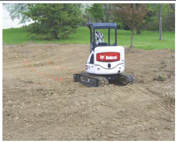
During excavation, check depths, slopes, and avoid soil compaction.
