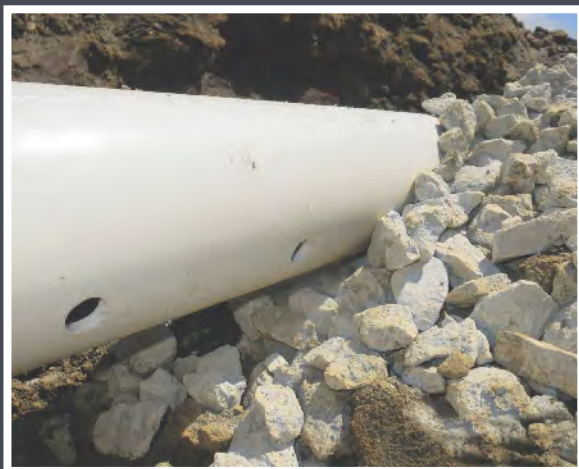
Place perforations downward onto drainage rock below
