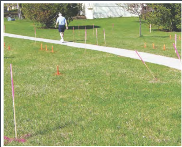
Stake bioretention garden prior to excavation.
