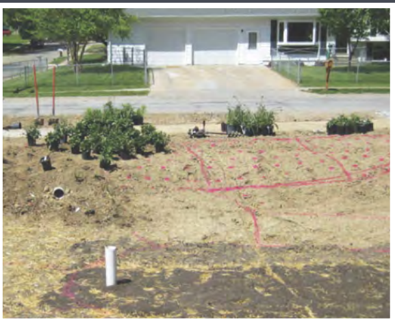
Use marking paint to define planting boundaries.
