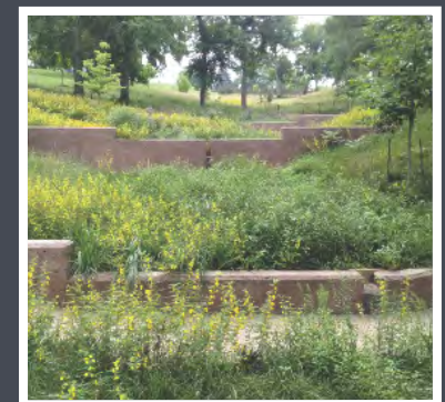
Seeded native grass and forbs in bioswale
