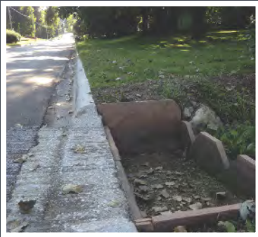
Flagstone pre-treatment with V-notch weirs in Saddle Hills Neighborhood
