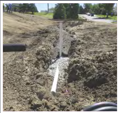
Creighton Prep infiltration cell construction
