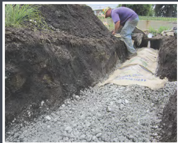
Mound drainage rock and separation layer upward
