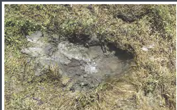
In-situ soil high in clay was tilled into the top 2 inches of the infiltration cell, clogging it right away
