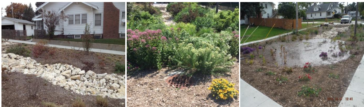
Figure 7. Photographs of the Benson East Gateway bioretention system showcasing the layered dry creek bed (left), strong summer growth (center), and inundated system (right).
