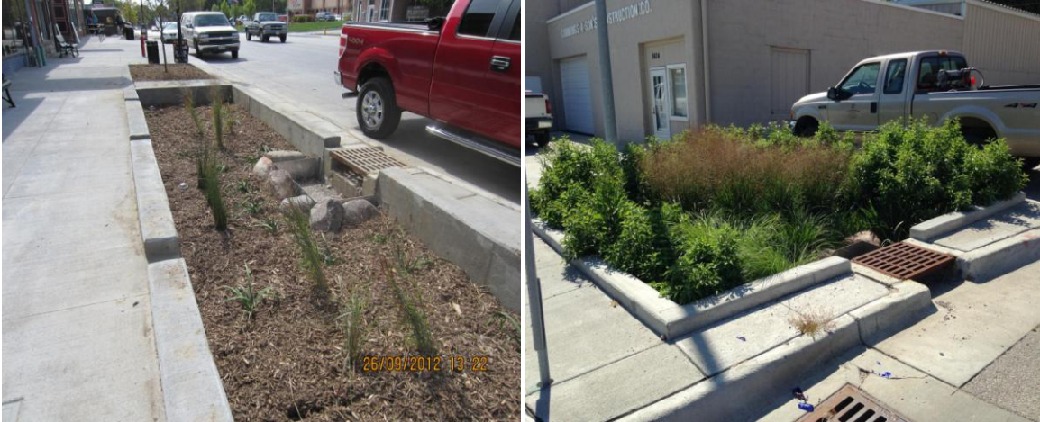
Figure 6. The east (left) and west (right) bioretention systems from the Florence Streetscape Project showing the stainless steel sediment traps pretreatments.
