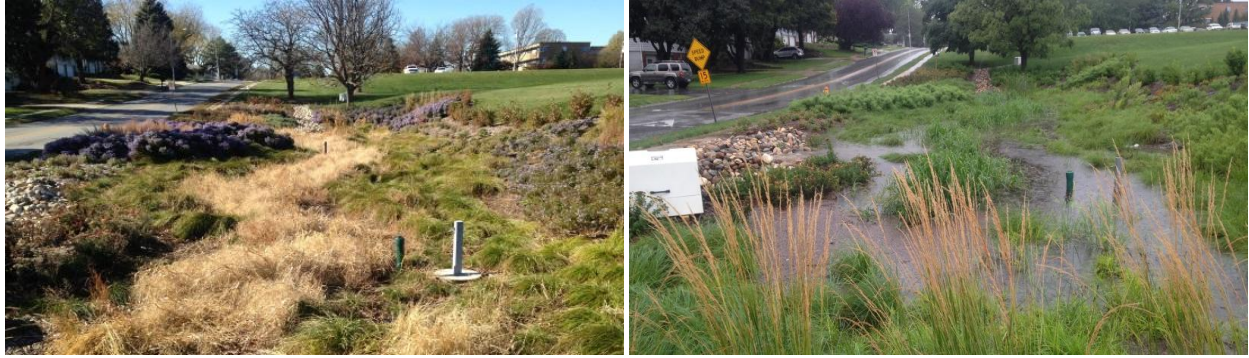
Figure 10. Creighton Prep bioretention system exhibiting summer growth (left) and inundated during rain event (right).
