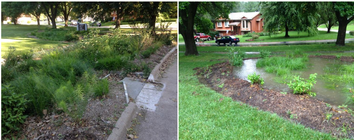
Figure 3. Photographs at Saddle Hills Park showing the east rain garden with utility box curb-well pretreatment (left) and the west rain garden fully inundated during a rain event (right).
