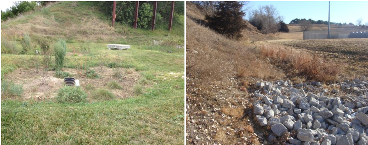
Figure 8. Photographs of the bioretention systems at the Under the Sink facility (left) and the bioswale that drains into bioretention system 1 (right).
